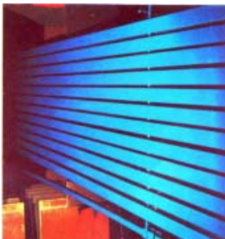
Installation horizontale de laquage
