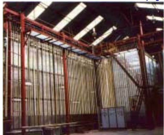
Installation verticale de laquage
